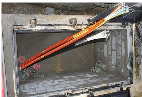
Figure 110: Bundles pulled in main duct
