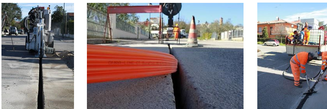
Figure 113: Micro-trenching deployment technique
