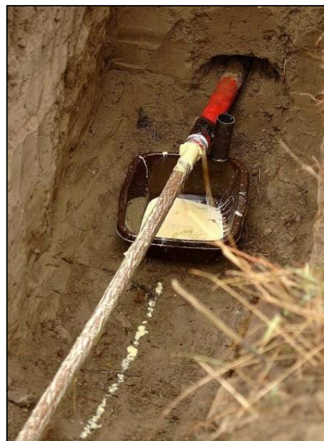
Figure 97: Cable de-coring
