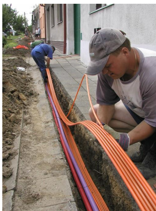
Figure 83: Deploying micro-duct infrastructure
