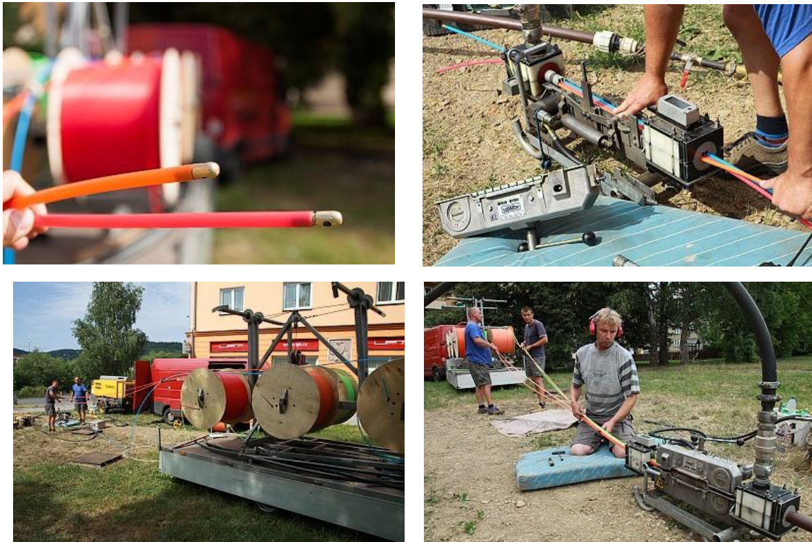
Figure 111: Air blowing of micro-ducts
