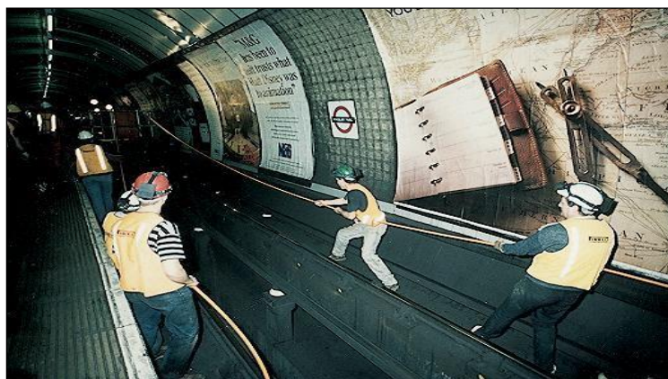
Figure 103: Cable installation in a train tunnel
