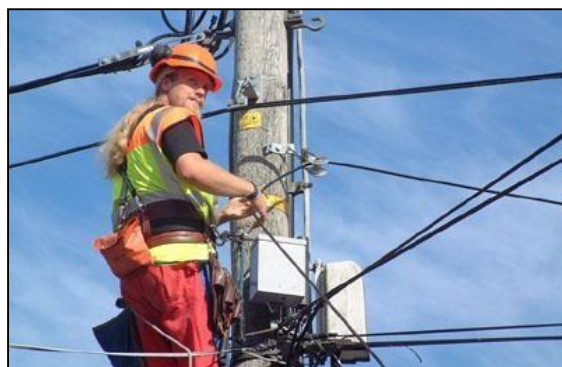
Figure 107: Aerial cable installation
