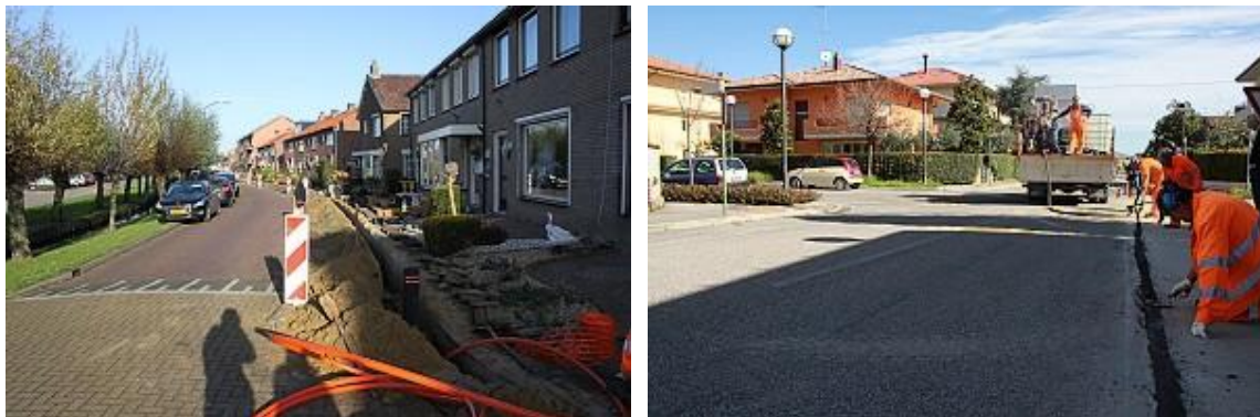
Figure 84: Conventional trenching vs microtrenching
