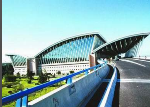
Shanghai, Pudong Airport, T2
